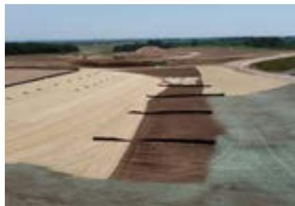
Silt Fence with Wooden Stakes
