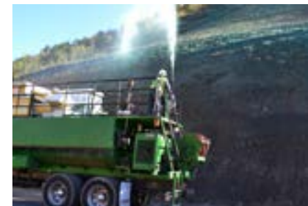
Hydromulch with Tackifier being applied
